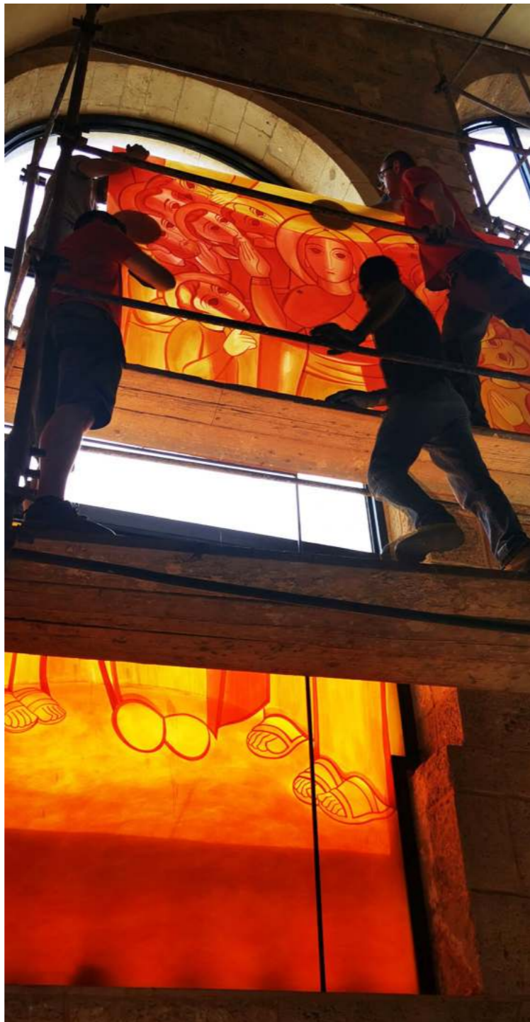
Installation of stained glass windows in Cathedral of Saint George Maronite, Beirut, Lebanon. (left page)
