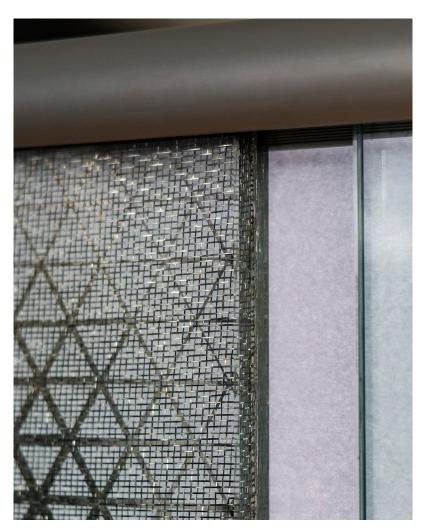
REMARK: Due to the metal meshes in the Multiple Weft Mesh models, it is also not possible to perfectly clean the lateral surfaces of the laminated glass.
